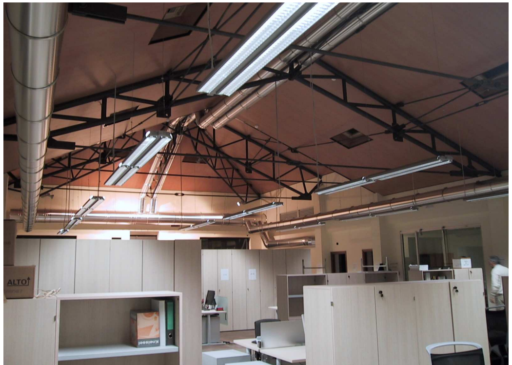
Open space - View of the welded tubular steel trusses
