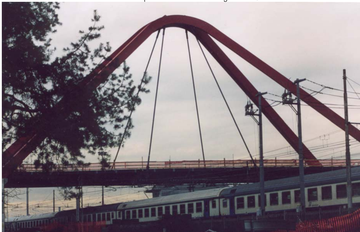
Rho - Road bridge with a 60 m span passing over the underlying railway line consisting of a bundle of nine tracks.
