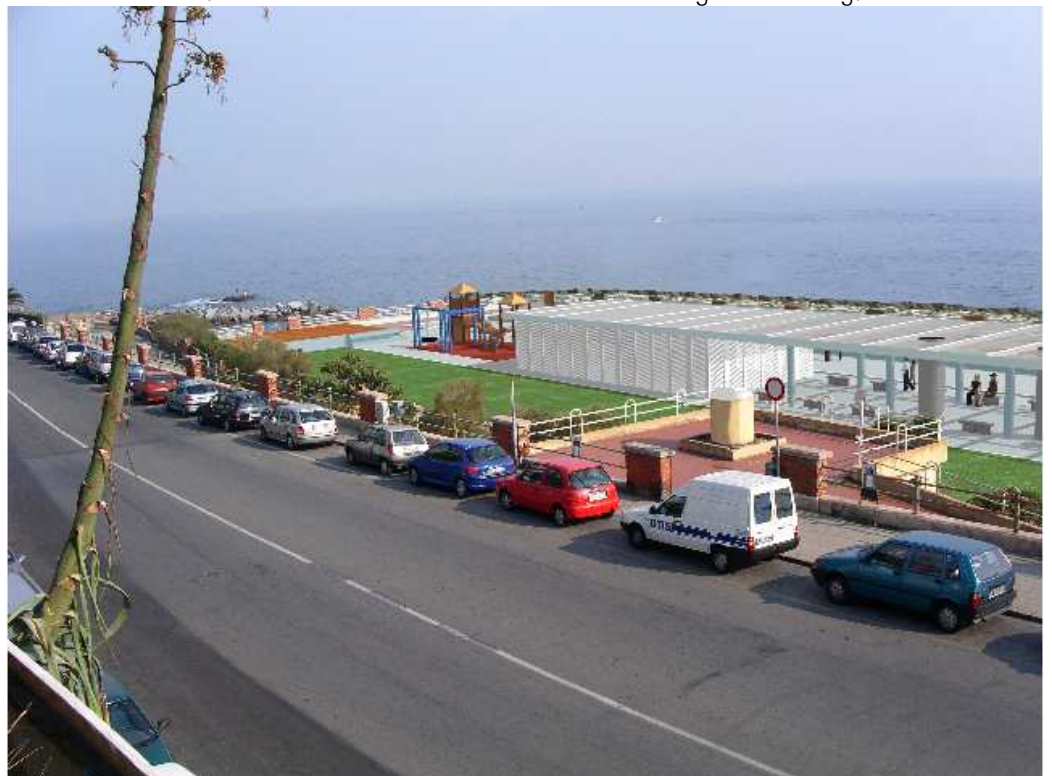
Photo-montage of the new roof arrangement at the Ge-Quinto wastewater management plant
