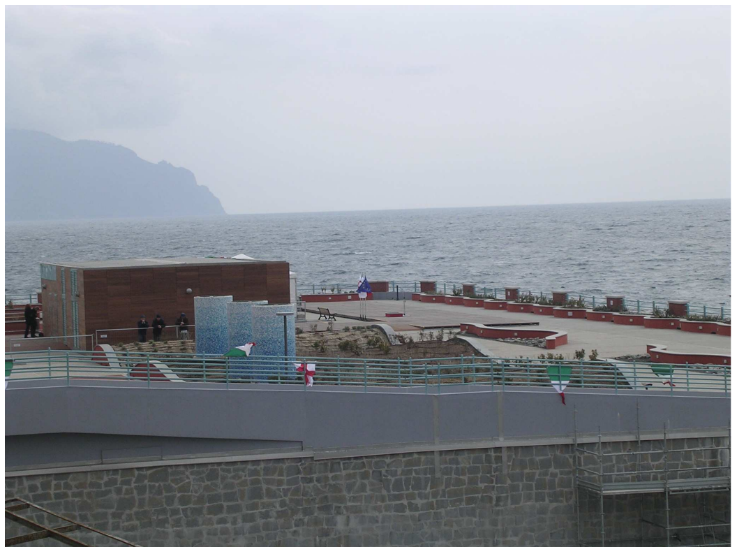
Photograph of the new roof arrangement on the day of inauguration
